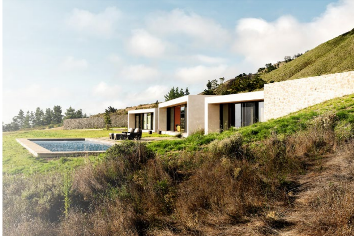
A net-zero house designed by Studio Schicketanz includes a natural landscape designed by Bernard Trainor of Ground Studio Landscape Architecture. Joe Fletcher
